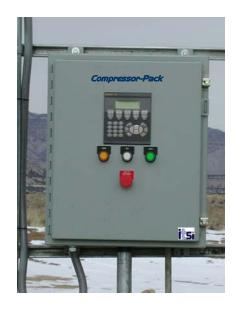
The Insight Technical Services, Inc. (itsi) Compressor-Pack is a Wellhead and Lateral Compressor Control Panel that is customizable to fit your needs, whatever they are. The Compressor-Pack was designed by itsi using the Control Microsystems SCADAPack32® PLC as our foundation. We have started with the SCADAPack32®, added our custom programming, and packaged the Compressor-Pack to be an off-the-shelf solution for your compressor automation needs.
