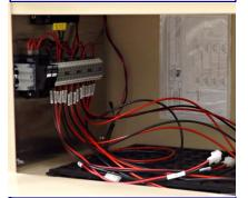
Quick disconnect from the power strip to the battery for added safety. Fused Input.
